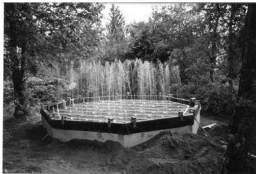
Sand filter squirt test during system construction.
