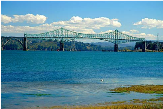
Bridge over Coos Bay, Photo by Gary Halvorson, Oregon State Archives
