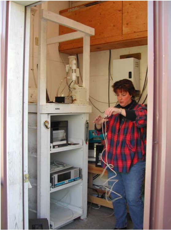
Jackie Brown – SWCAA performing maintenance on equipment at Wishram – December 3, 2003
